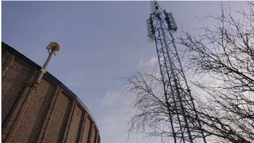
Figure 1.5: Station 0MOL and the newly installed radio mast.
