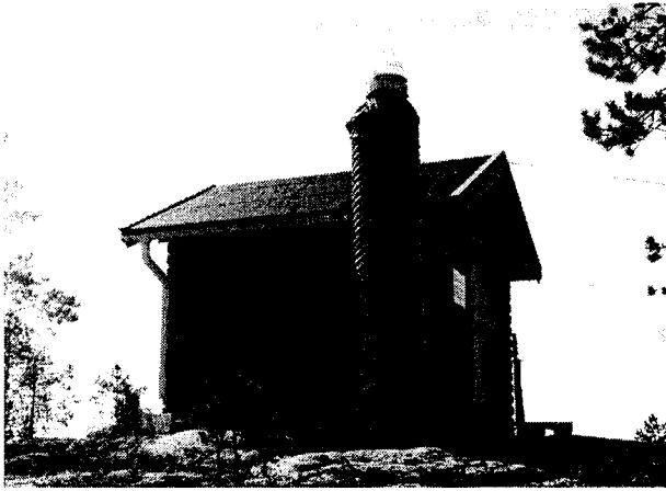
Figure 2. Reference station at Skellefteå.
