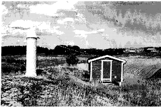
Figure 4: The SWEPOS station at Vänersborg with a SWEPOS standard pillar and conical radome.
