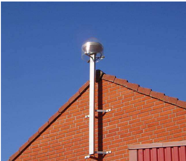
Figure 3: The SWEPOS station Smygehamn is a station with a roof-mounted GNSS antenna mainly established for network RTK purposes belonging to Class B.
