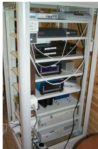
Fig. 5 Instrument rack on the SWEPOS-stations
