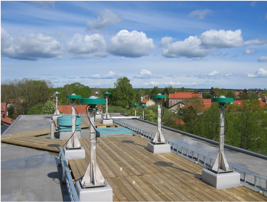
Figure 3.16. The antenna test field on the roof of the Lantmäteriet building in Gävle.
